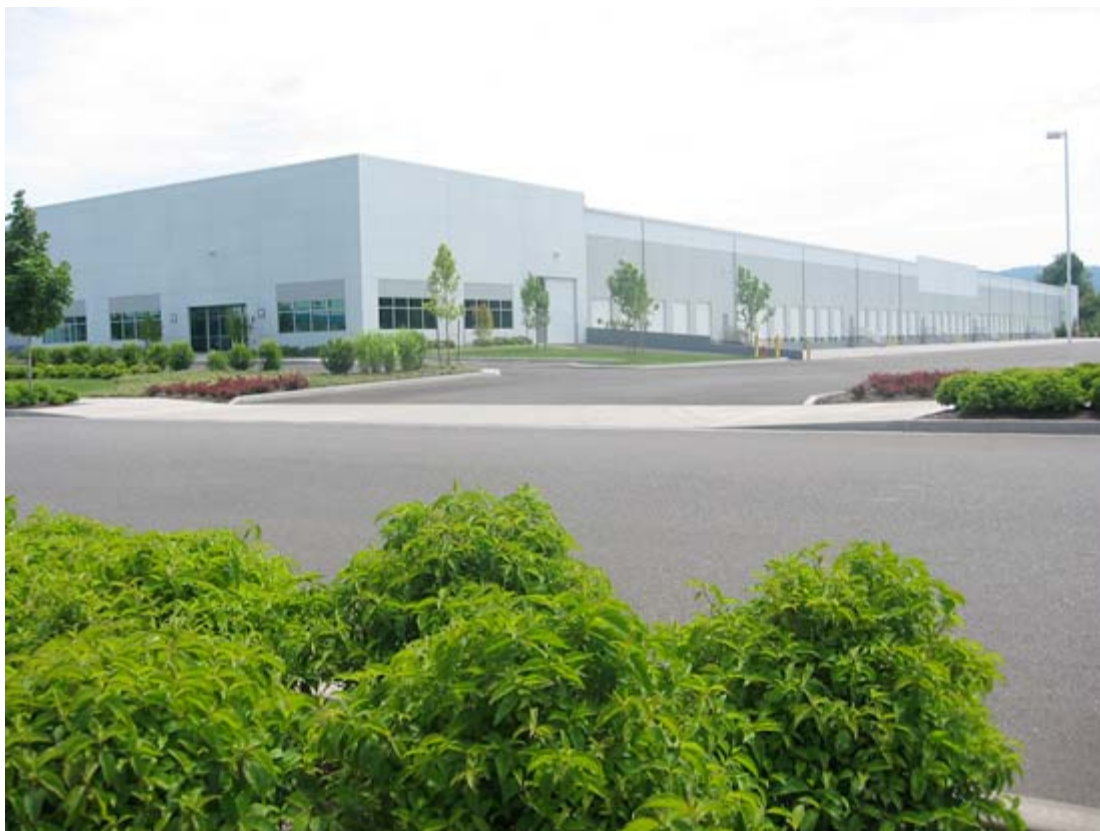
Solaicx Oregon Manufacturing Facility
